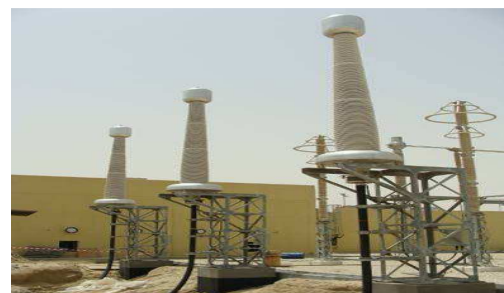
Figure 6: 400 kV Termination under construction
