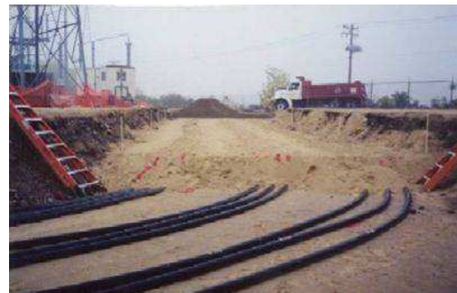
Figure 18: Installation of 400 kV XLPE cables
