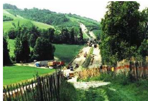
Figure 17 : cable route at site
