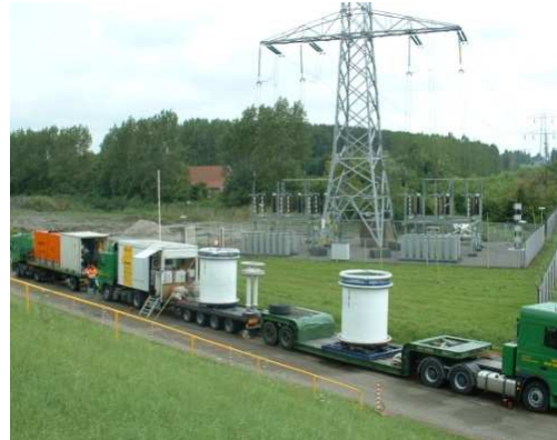
Figure 7: Test after installation in proximity of an overhead – underground transition compound
